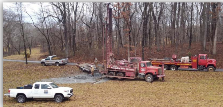
Water Supply Well Installation
