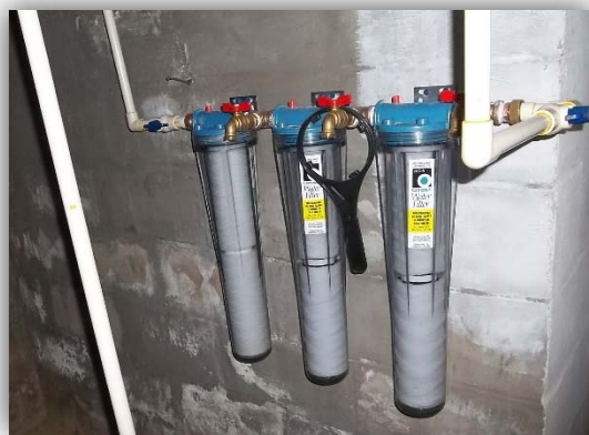
Typical Residential Filter Installation
