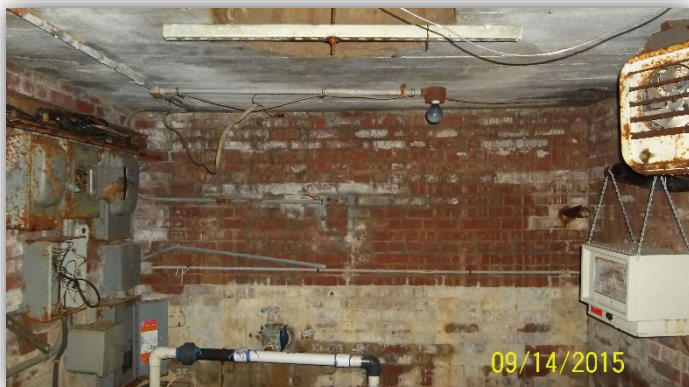
Initial Wellhouse Condition
